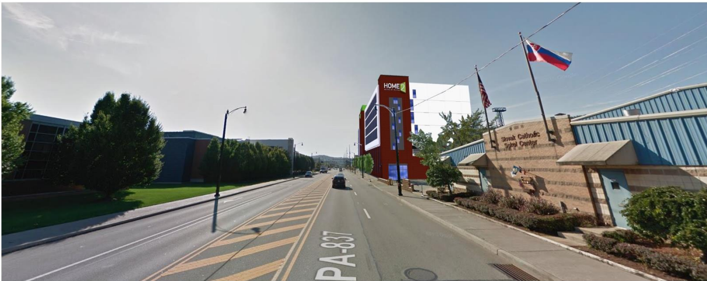
APPROACH FROM NORTH-WEST
